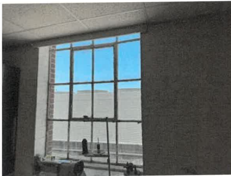
Painted Metal Windows were found to utilize lead-based paint.
