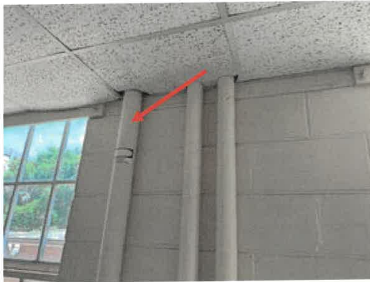
Labeled Aircell Pipe Insulation
